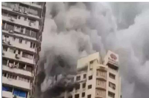
Photo-5-Kamal mahal-Under fire
