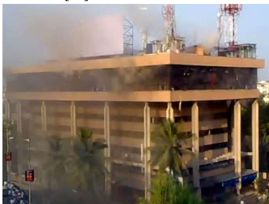
Photo-3-Carlton tower-Under fire
