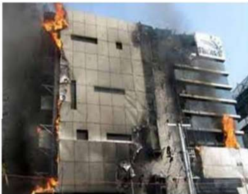
Photo-1 –AMRI Hospital- -under fire
