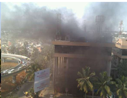
Photo-4-Carlton tower-the extent of smoke
