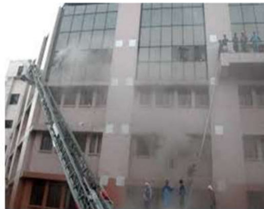
Photo-2 -AMRI Hospital- -Glazed Facade
