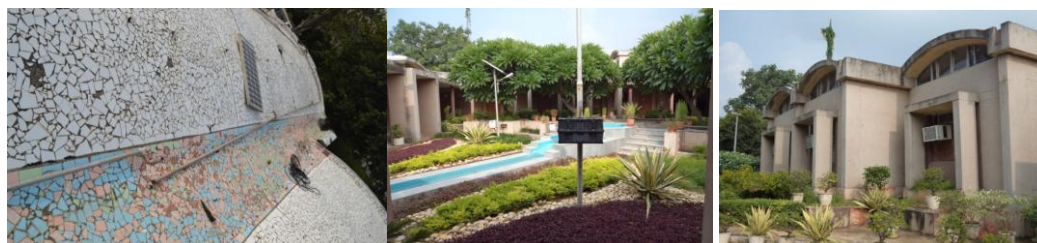
Fig. 4- (a) Use of reflective material in roofing (b) Use of water in courtyard (c) Openings for lighting (Source: Ref. 4)
